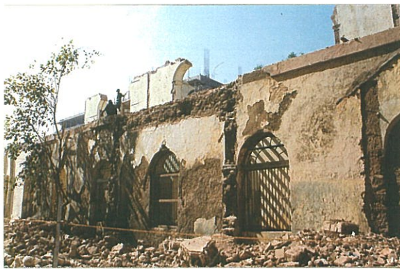
Demolition of Old Collector's Office
