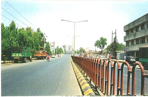
Implementation of road widening program
