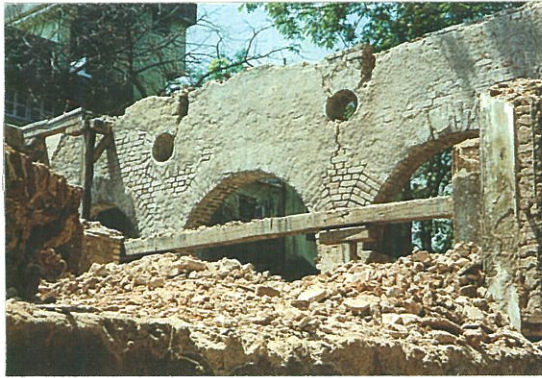
Demolition of B. J. High School
